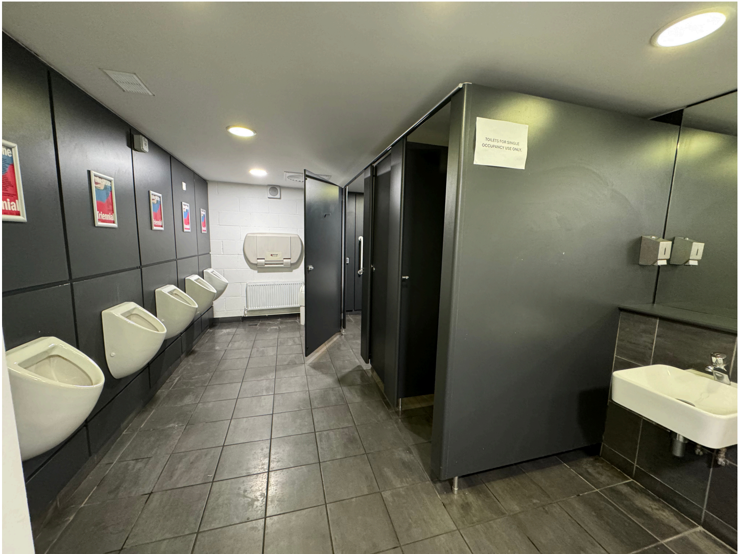
The accessible toilet is in the far corner
